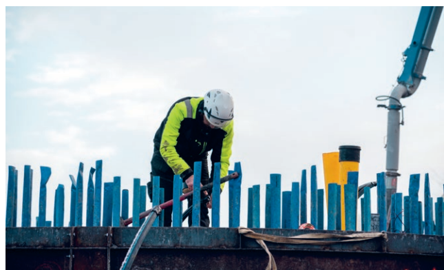
Intensive work with the foundations for Tjárnäs took place during autumn.
