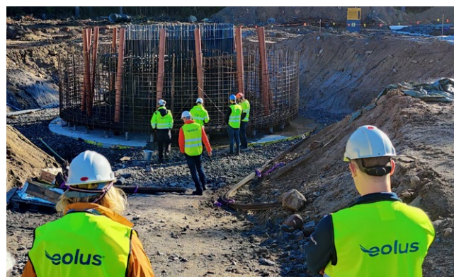
The foundations for the Rosenskog project were cast during autumn 2022.
