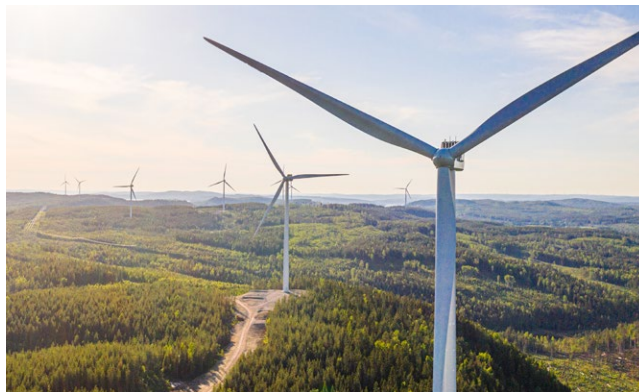
Onshore wind power is still the fastest and most cost-efficient technology to build. The Nylandsbergen wind farm in Sundsvall was completed in 2019.
