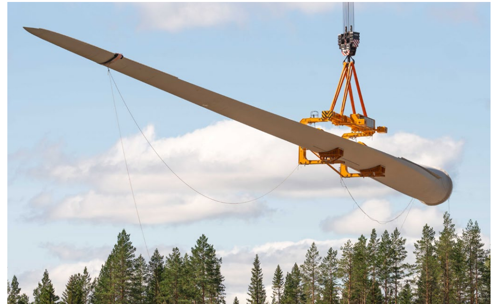
About 90% of a wind turbine can be recycled, but the rotor blades represent a challenge. A lot of progress has been made in recent years, however, and a chemical process can be used to break down the epoxy-based rotor blades. Turbine manufacturers have also launched recyclable blades.
